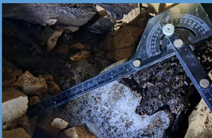
Photo1: Condition of the residual glacial deposit (Survey April 2025). Detail of the cavity floor showing the disappearance of the historic slab, reduced to a thin layer of interstitial ice covered by rock debris. (Ph M. Mugione).
