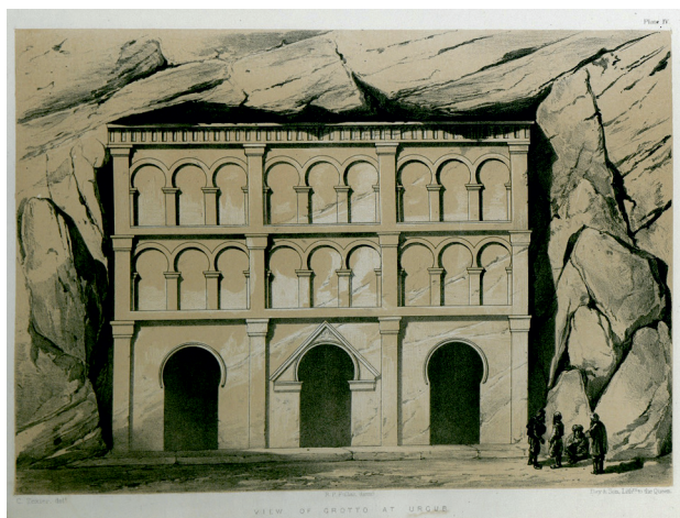
Fig. 2. Engraving by Texier showing the facade of a rock-cut structure (Texier 1839)
