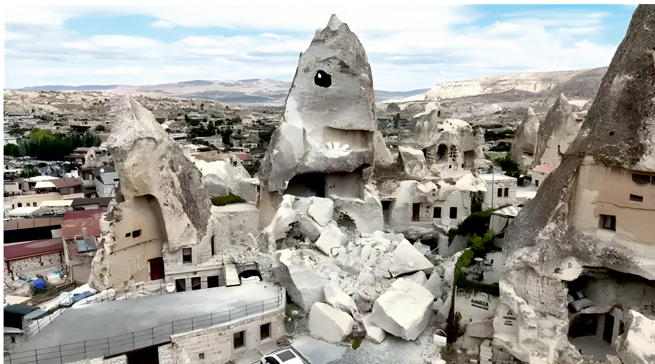
Fig. 5. Göreme, collapse of a fairy chimney at Sept. 20, 2025 (photo Anadolu Ajansı)
