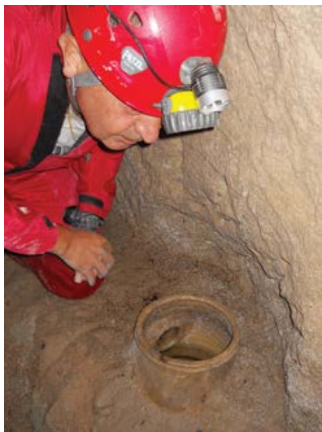
Fig.8: jar used as a utility hole on the terracotta pipes (photo E. Gilli).
